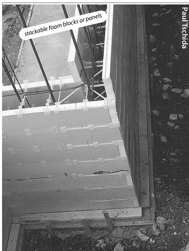
Insulated concrete forms contain poured concrete and provide excellent thermal resistance for basements and home walls.
